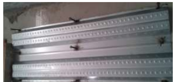
Fig2 Specimen before casting concrete
